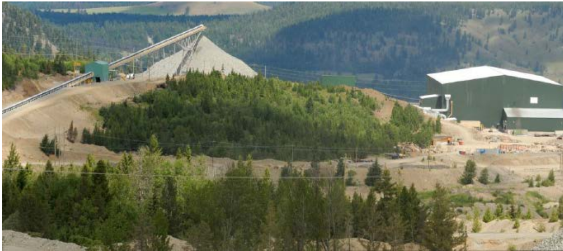
Figure 14 - Original stockpile conveyor configuration with concentrator building on far right hand side
