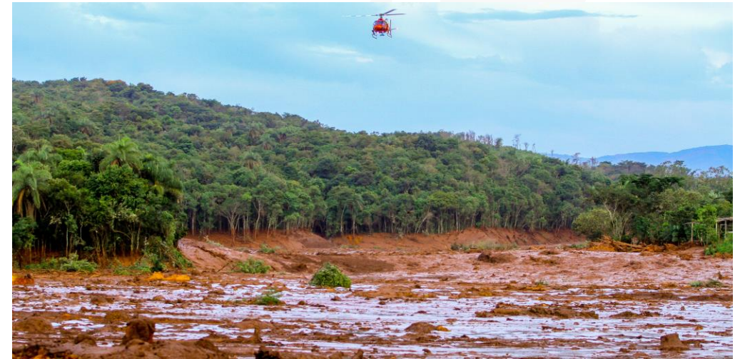
Brumadinho Dam Failure in Brazil
