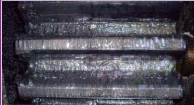
Pinion Gears with Asphaltic Type Lube
